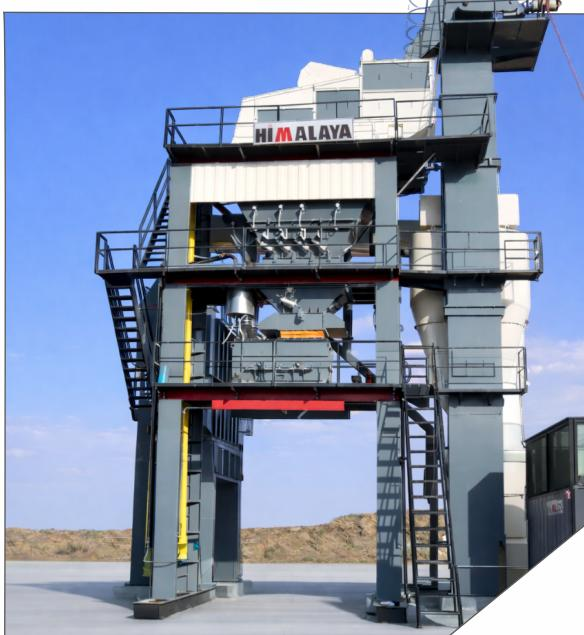
The batch tower is equipped with a fully enclosed inclined liner vibrating screen fitted with high-quality screen meshes to ensure efficient and reliable screening performance. The screen is supported on a duplex spring system and driven by two six-pole, maintenance-free vibratory motors, providing smooth and consistent operation.
