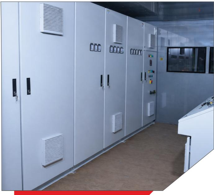
All HBM series plants are provided with a fully computerized, air-conditioned control cabin featuring an onboard electrical power control console and distribution switchboard. Fully automatic process and sequence control comes as a standard offering. User-friendly software integrated with a PLC-based main machine interface ensures high reliability and consistent top-level performance.
